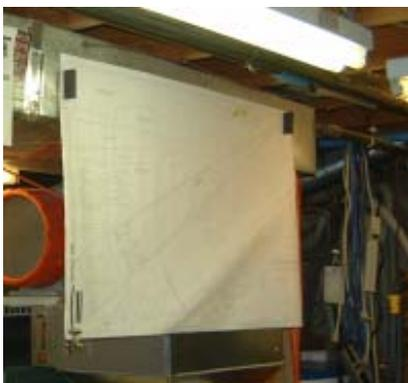
Heavy duty magnets suspend plans from the ductwork.
